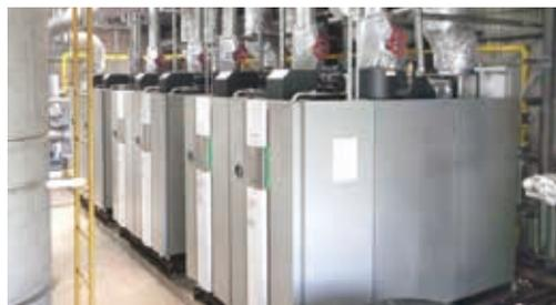
High-efficiency, energy-saving gas boiler facilities (Kashima Plant-West)
